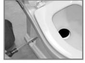
bowl is clear, turn screwdriver or socket wrench clockwise to return flush ball to original position.
