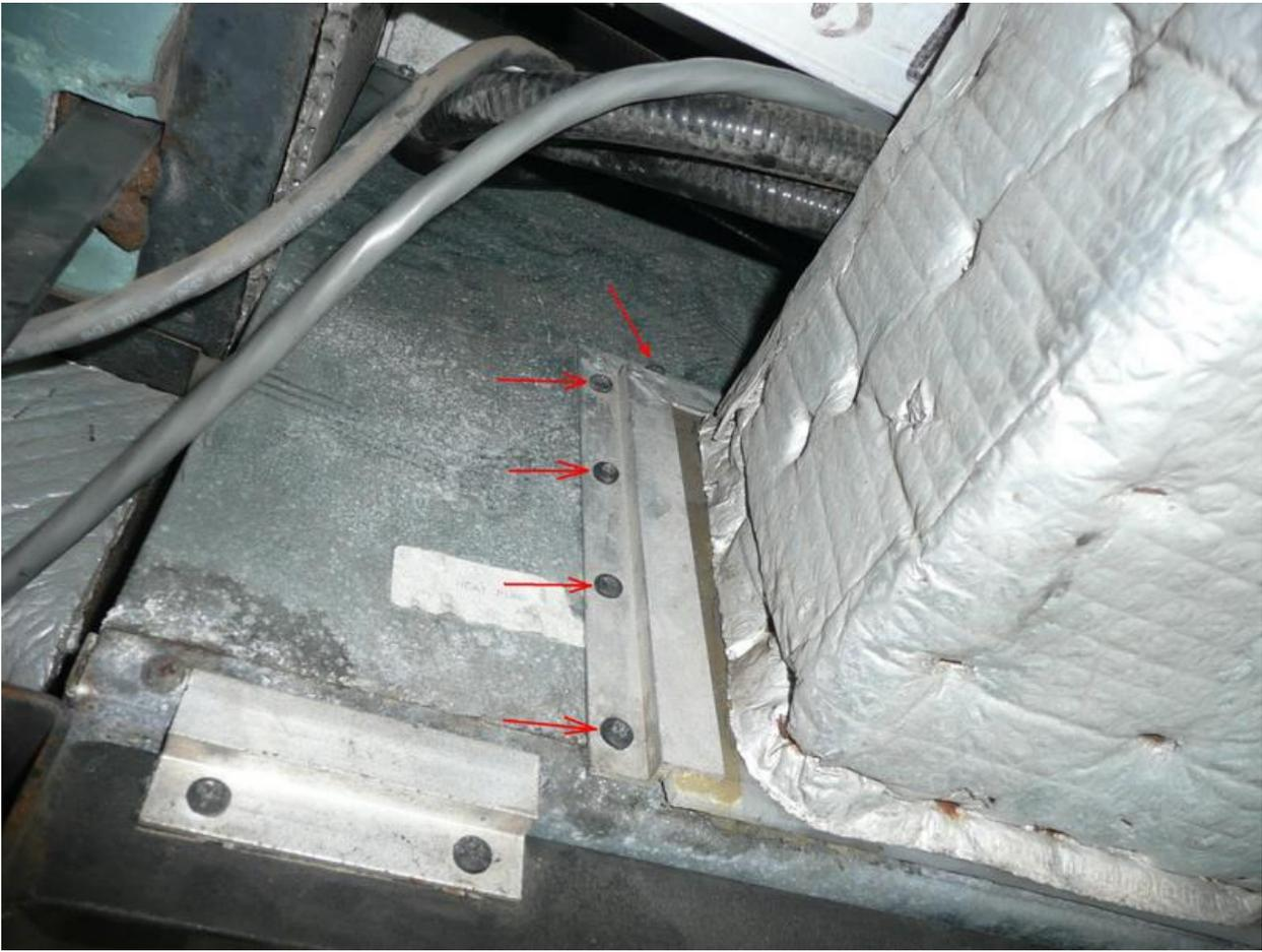
5. Remove the 5 screws on the right side of duct. A short 6" screw driver is useful on the top 3 screws. Have a helper hold the power cables back out of the way to aid access to screws.
