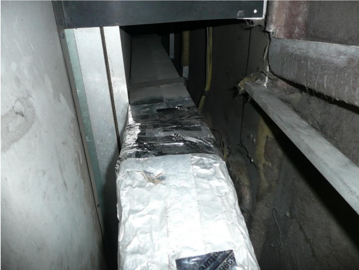
8. Use a bungee cord to hold duct back about an inch so the foam seal is not torn off.
