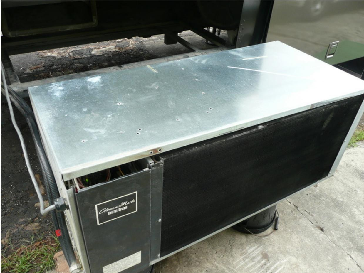
12. Take off the top cover by removing the approx 28 screws.
