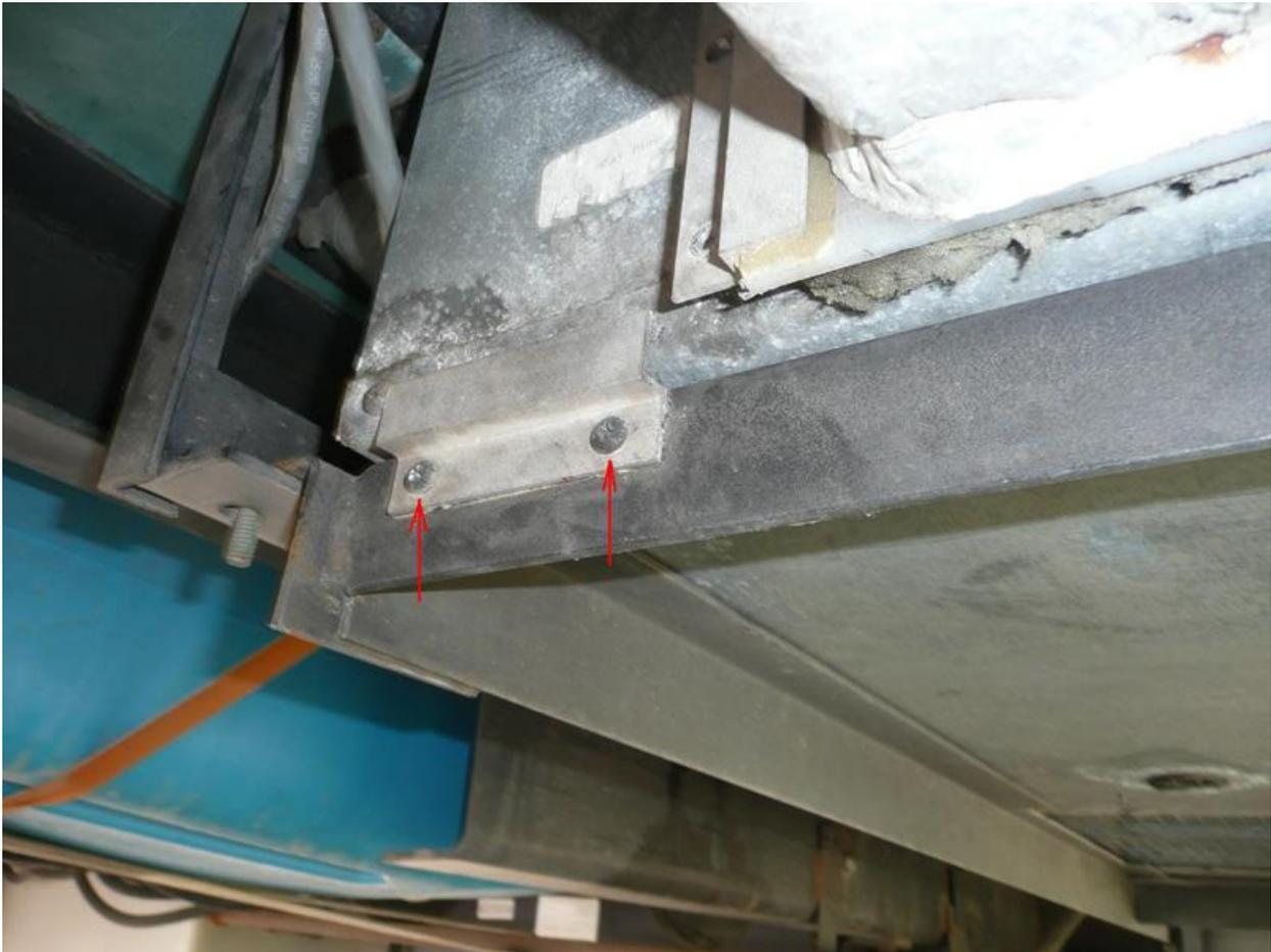
7. Check the seal of the aluminum tape about 1.5 foot up the duct work. In my case the whole 90 deg elbow fell to the ground because the alum tape adhesive had dried out. I had to cut about 3 in of alum tape off and re-taped with "Venture Tape". Venture Tape is very expensive (\$35/roll), but it is designed to hold duct joints permanently in very hot/cold attics.
