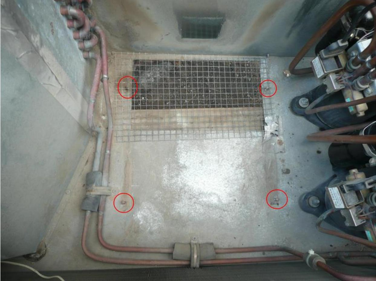
21. Use reverse procedure to re-install the blower assy. Use a little sticky butyl rubber on the nut to hold in the 7/16 socket to get the nuts started.
